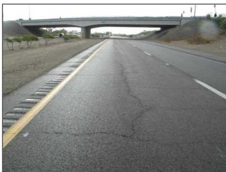
Figure 7. NMVCCS Case No. 2007-078-071 shoulder width
